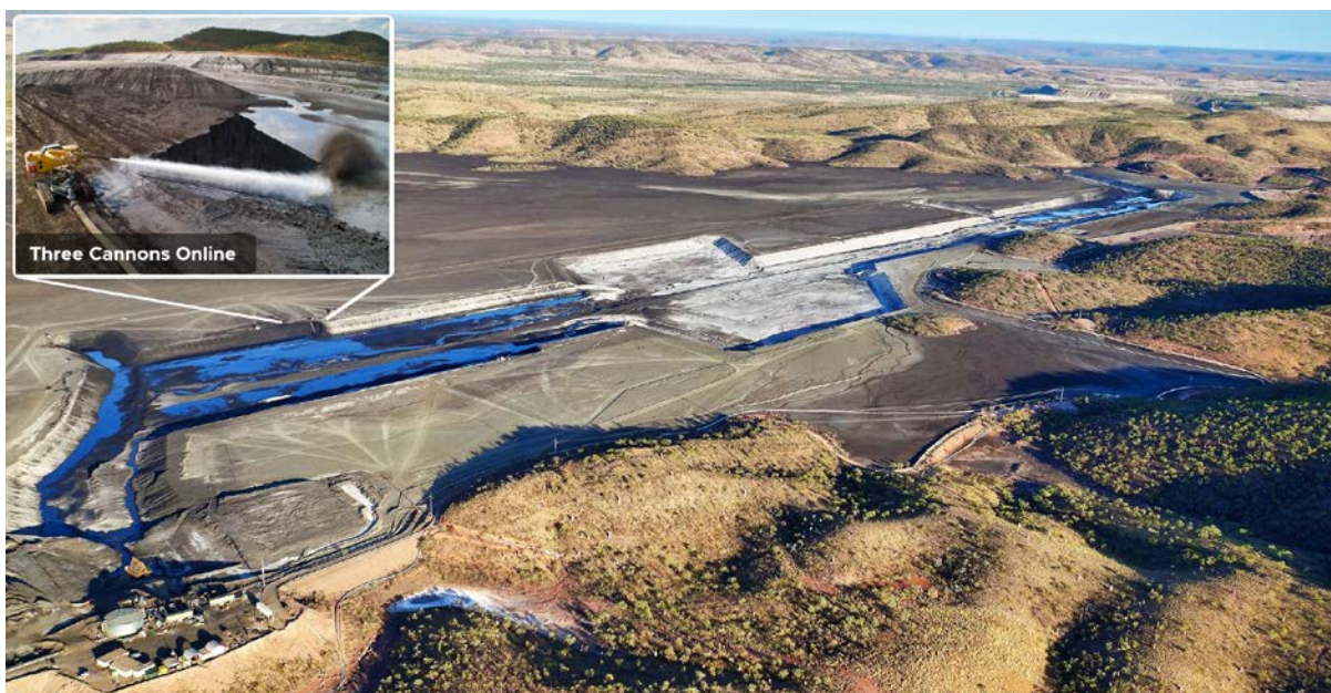
Figure 5: Overview of hydraulic mining progress at the Century
