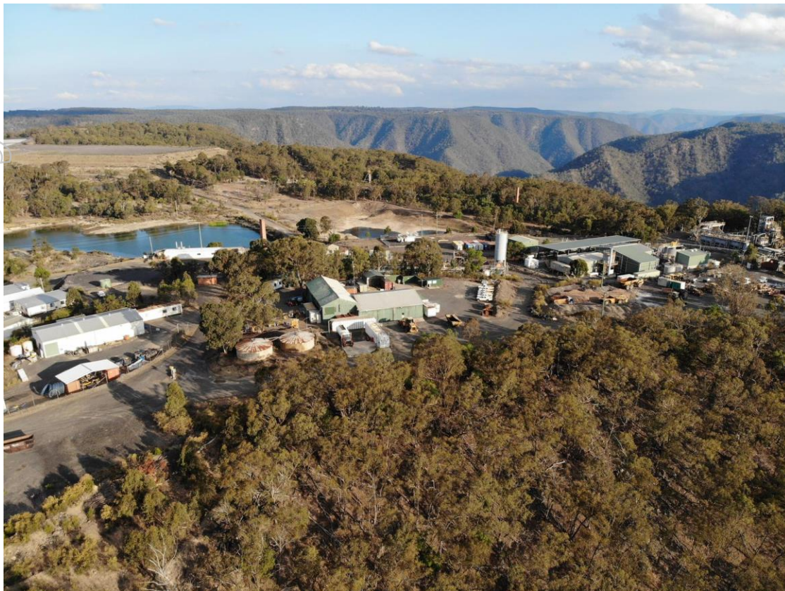
Figure 1 Hillgrove Gold Mine showing processing infrastructure and layout
