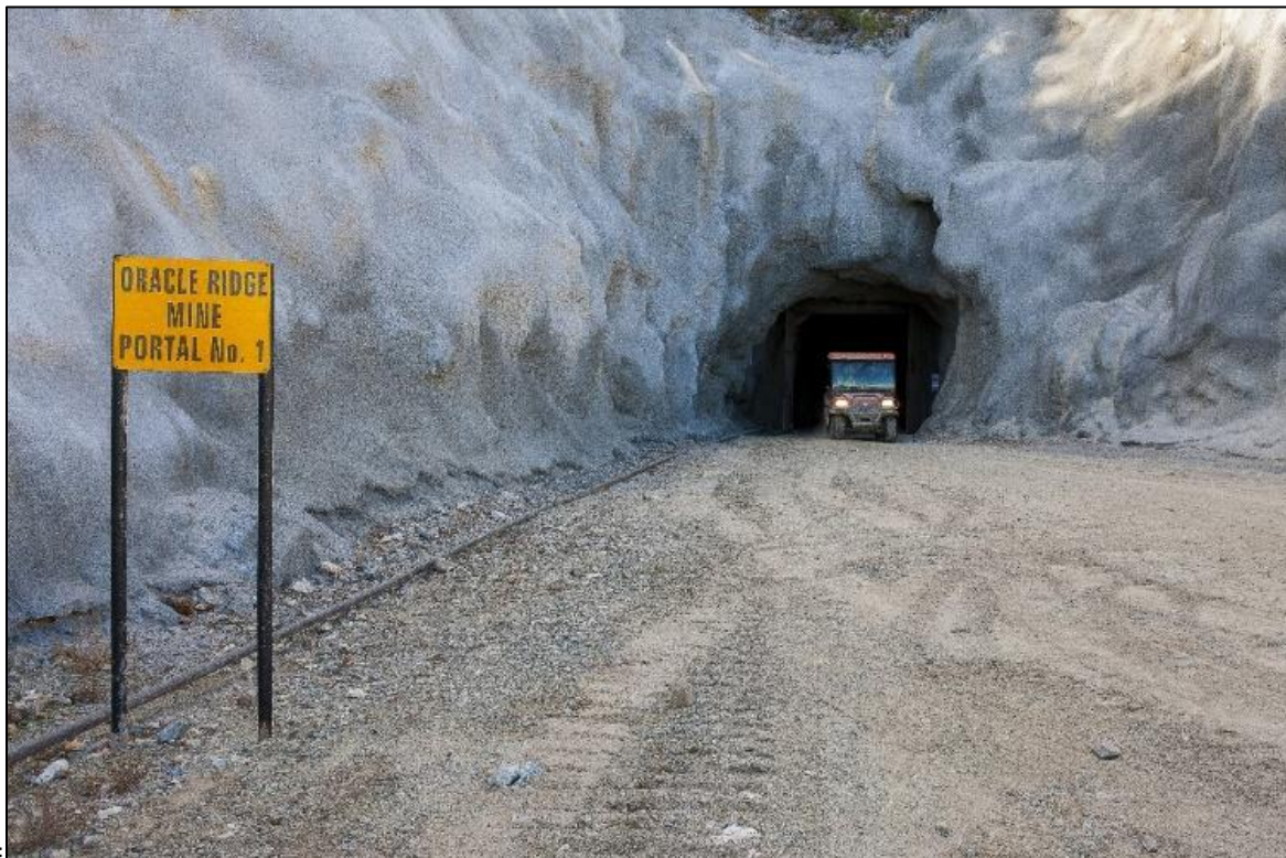
Figure 1 Oracle Ridge mine - 5900 portal
