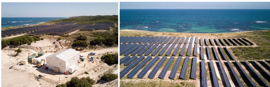
Garden Island Microgrid
