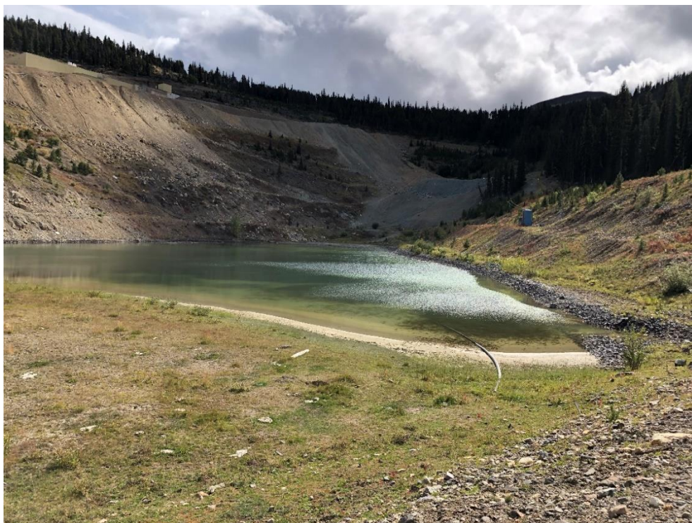
Figure 10 – Blackdome Tailings Storage Facility
