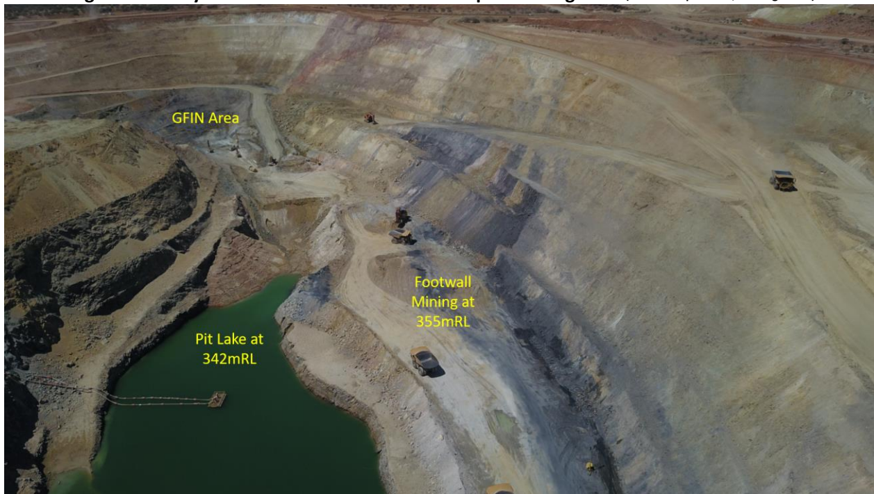
Figure 2: Gilbey's Pit Lake level ~12m below deepest mining level (as at 30 September, looking north)
