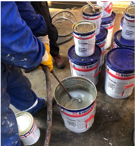
Figure 6 Mixing of epoxy coating system.
