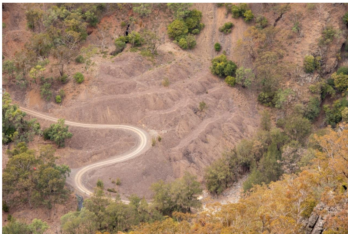
Figure 2 Bakers Creek Waste Rock Dump (August 2019)
