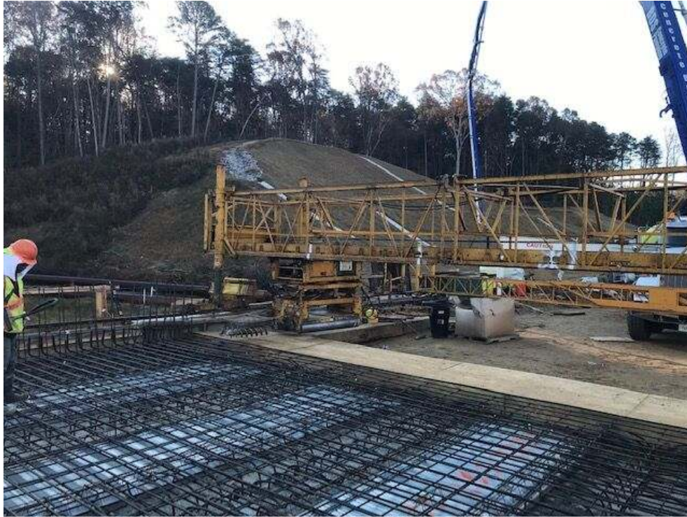
Figure 2. Bridge over Little River showing re-enforcing steel included in bridge decking
