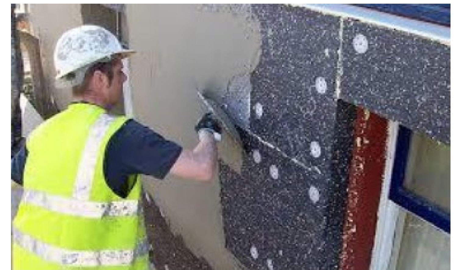
Installing Flame Retardant Foam
