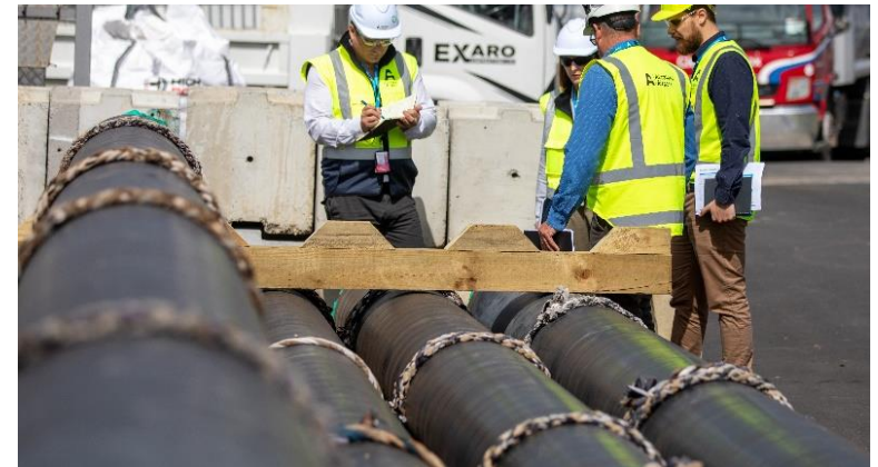
Airfield fuel pipeline upgrade
