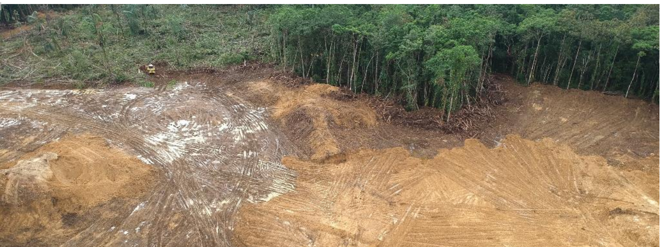
Figure 4: Plant Site Clearing
