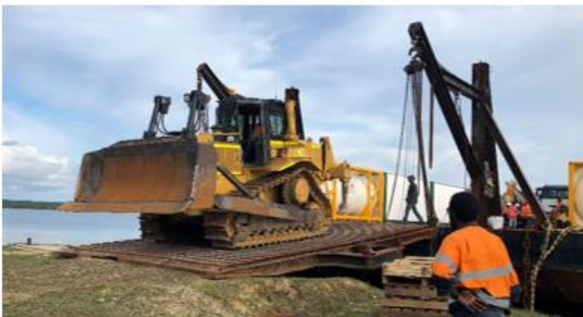
Figure 2: Equipment Mobilised to site by Barge
