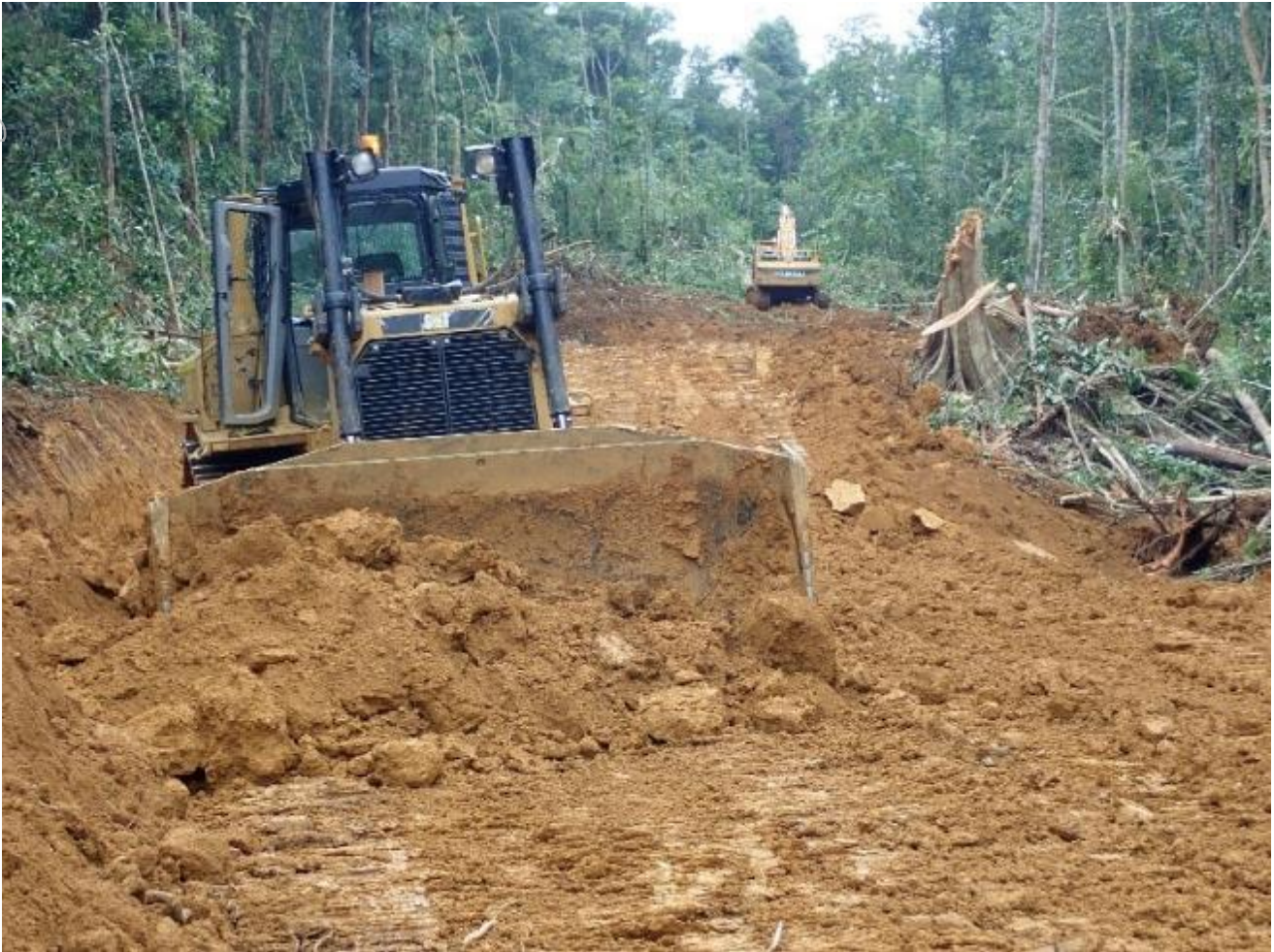
Figure 5: Wharf road pioneering works
