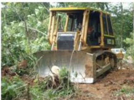
Figure 6: Clearing activity for village
