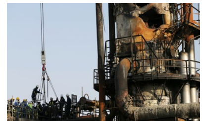
Damage caused by the September 2019 drone attacks on Saudi Arabian oil facilities
