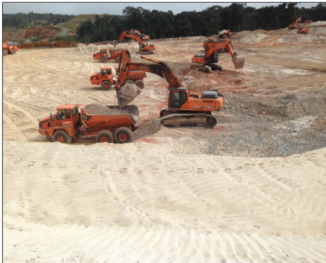
Mining at Hicks 4 in January 2020
