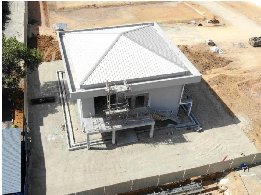
Figure 2 – Electrical substation construction progress March 2020 (North aspect)
