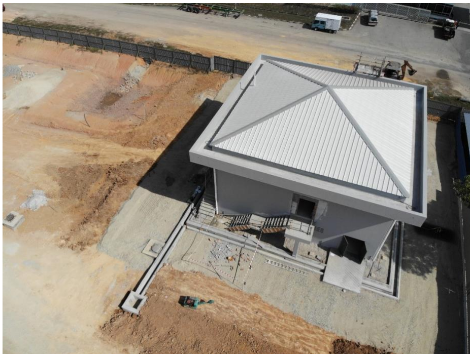
Figure 4 – Electrical substation roof completion March 2020
