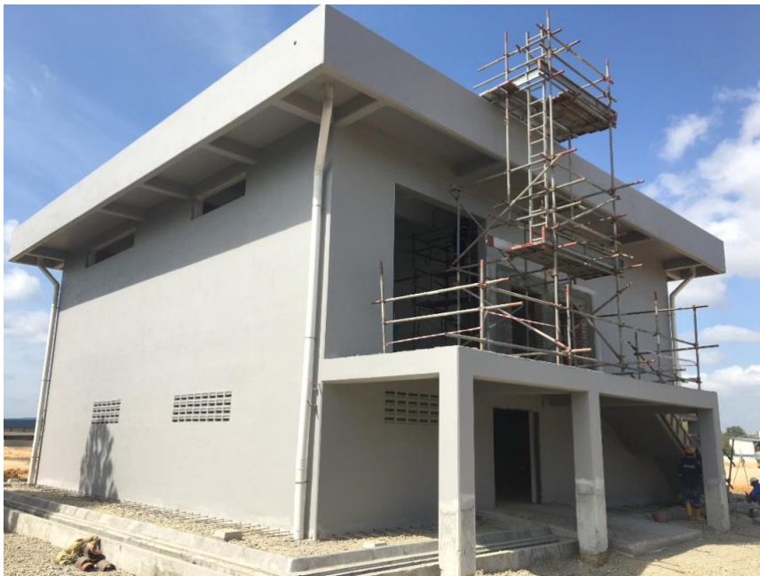
Figure 3 - Electrical substation construction progress March 2020
