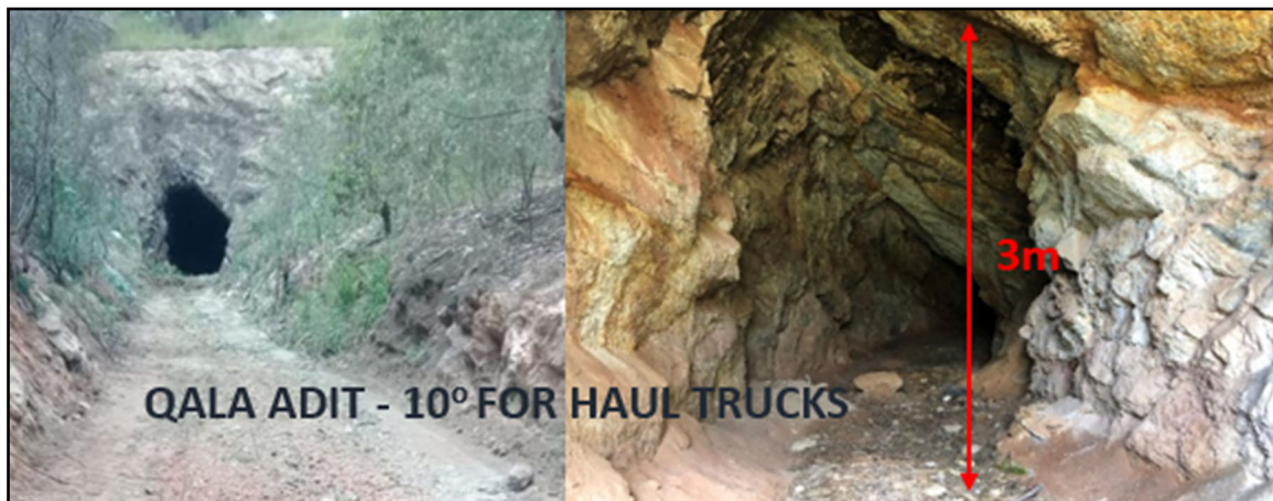
Image 2: Qala Adit will provide access to the Kimberley East underground target.
