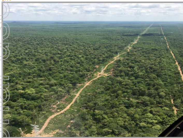
Figure 3 | Aerial View Powerline Towers and Corridor 15 km from site
