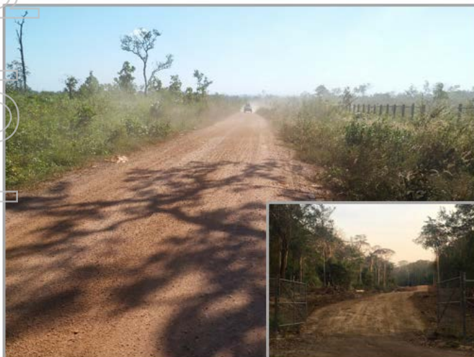
Figure 5 | New Road Construction
