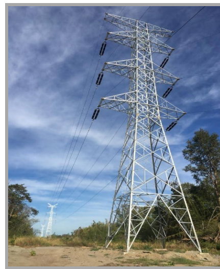
Figure 4 | Erection of towers to supply grid power at Okvau
