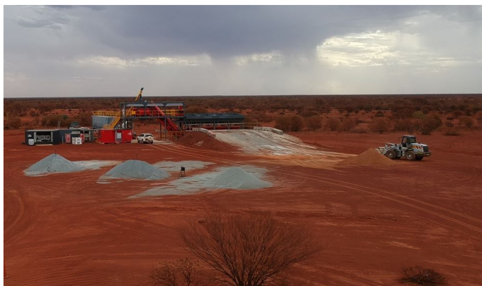
Concrete Batching Plant
