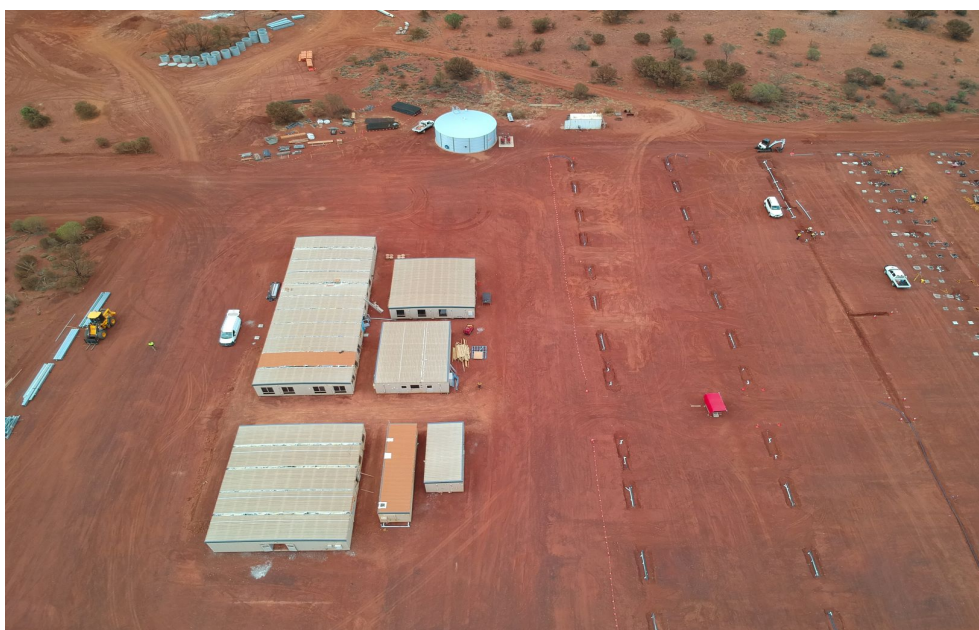
Installation of accommodation village
