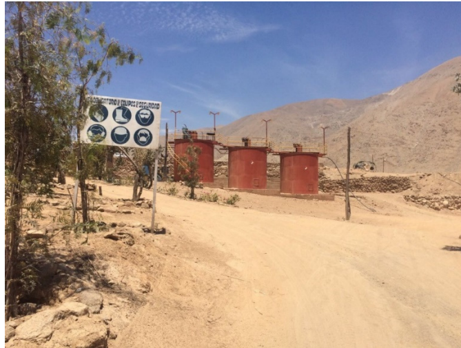
Photo 1: Haul Road entrance to existing Chimu Gold Plant
