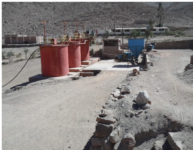
Photo 2: Leach tanks, ball mill & Switch-room: with accommodation block & Laboratory in the background: Chimu Gold Plant
