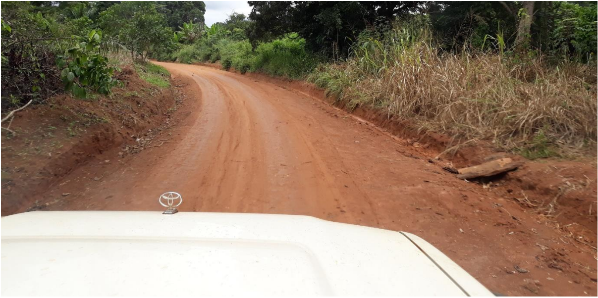
Figure 9: A section of reconstructed internal access road
