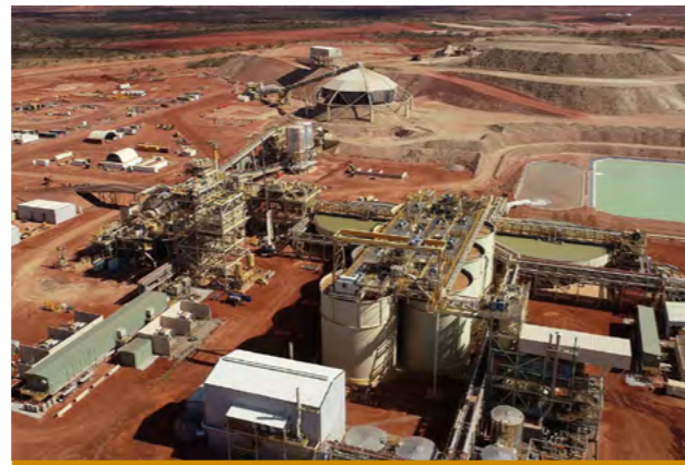
Aerial view of Gruyere Process Plant
