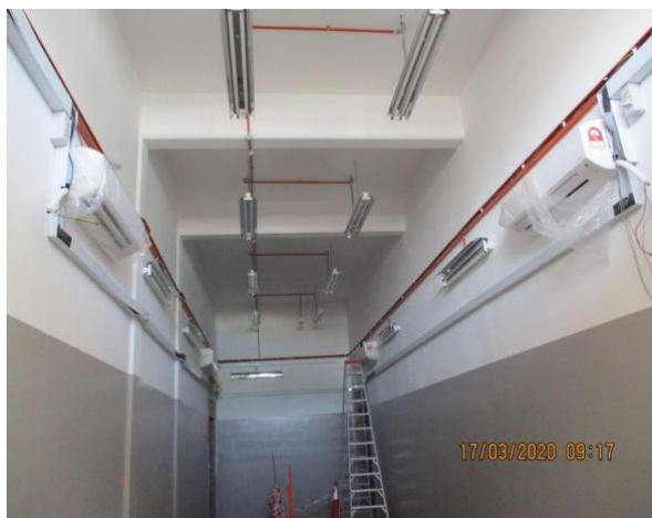
Figure 1 – Substation internal finishing
