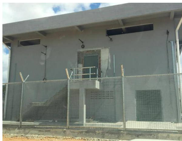
Figure 2 – Completed substation structure, fenced
