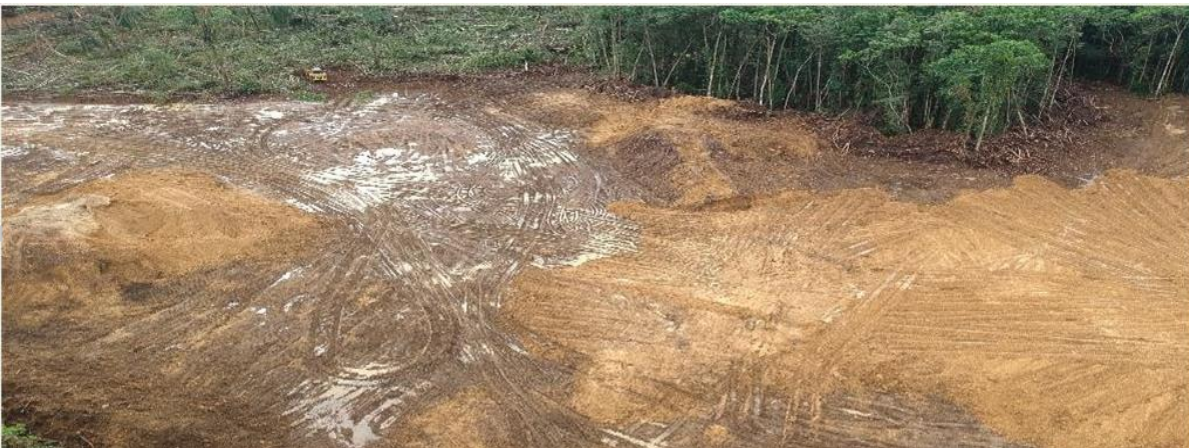
Figure 7: Process plant site cleared as part of the Civil Works Program
