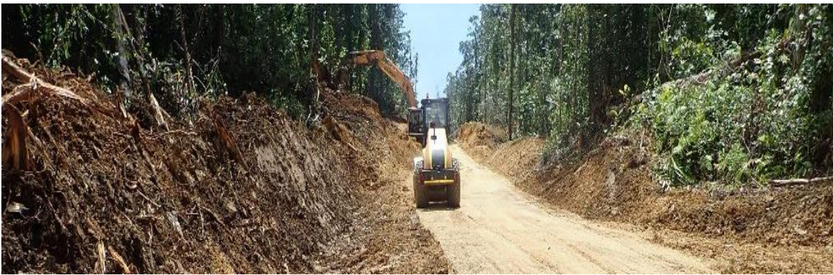
Figure 8: Road clearing activity on the Woodlark Island
