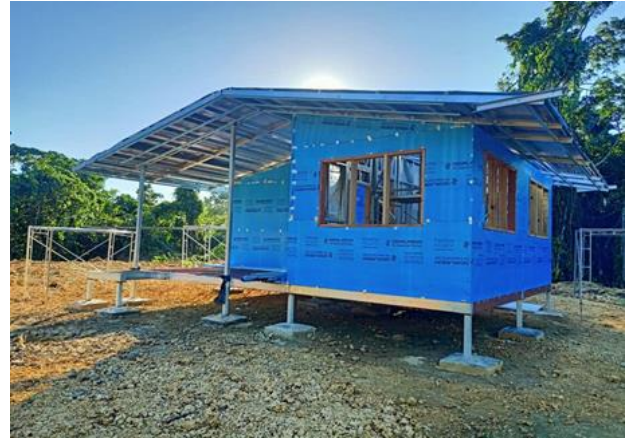
Figure 11: New house under construction
