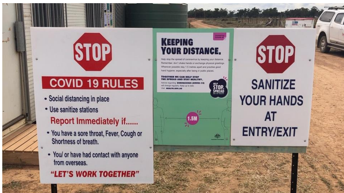
Figure 1. JSP Construction Site
