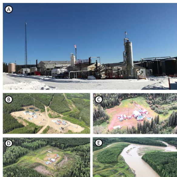
Figure Two – Tommy Lakes Field A. Tank storage, liquids handling facility and West 1 compressor, B. Field office, control room and camp facility, C. West 2 Compressor, D. West 1 Compressor, E. Location where the Tommy Lakes pipeline crosses underneath the Sikanni Chief River.
