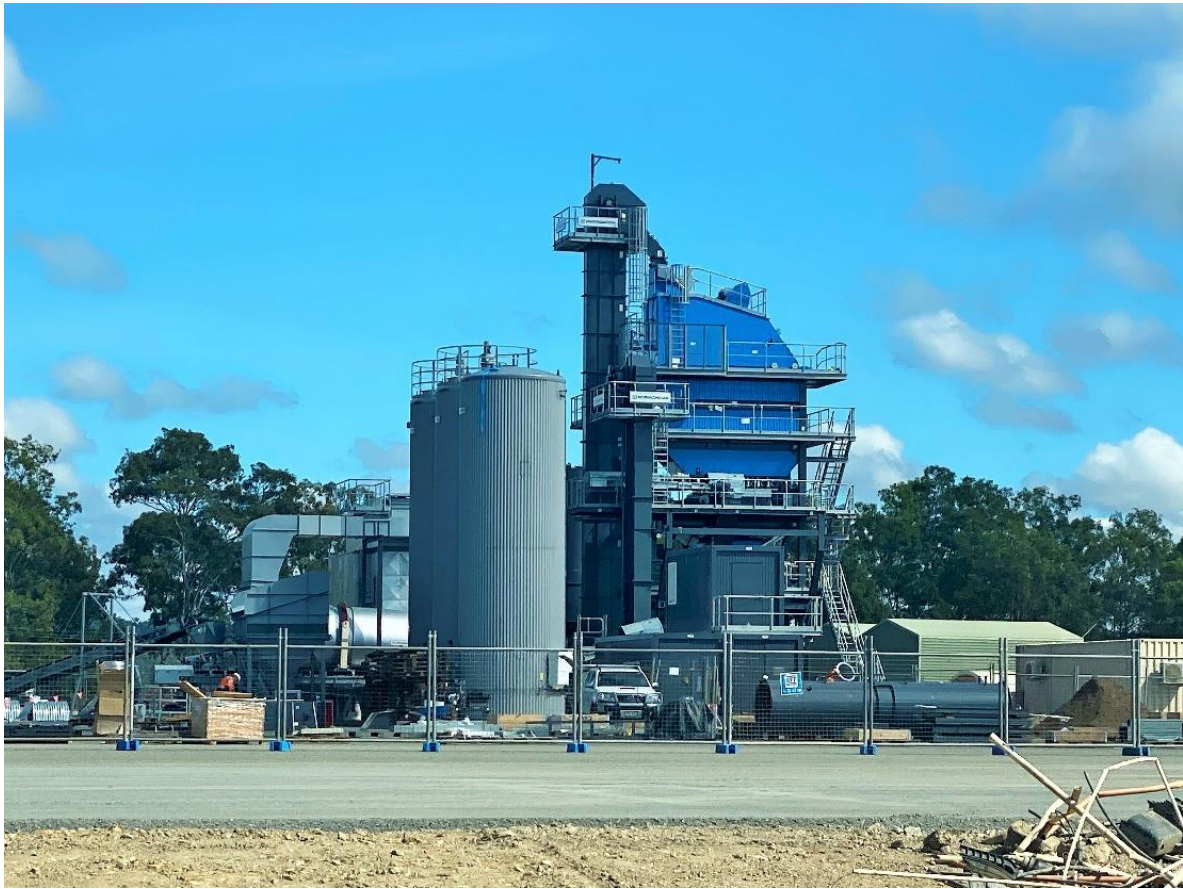
Aussee Road Services new asphalt plant 30 th March 2020 Source: Company
