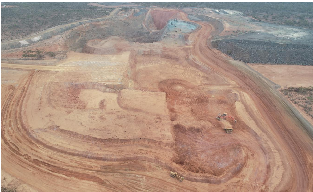
Figure 1: Commencement of mining at Karonie South during the quarter
