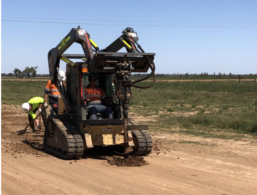
Figure 1. Construction activities underway at JSP, located near Forbes, NSW.
