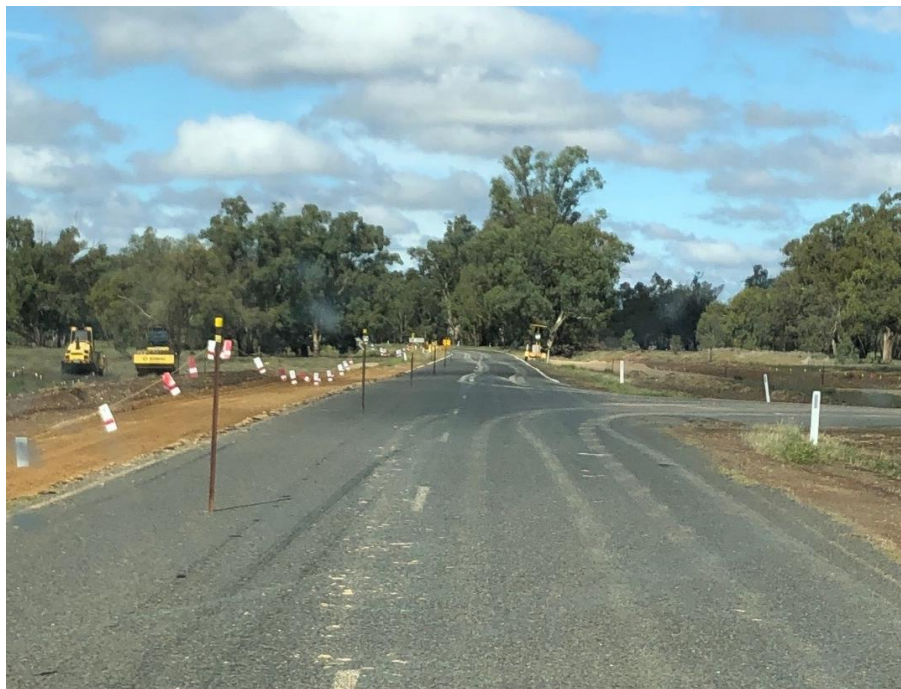
Figure 2. Road works underway at the entrance to JSP.
