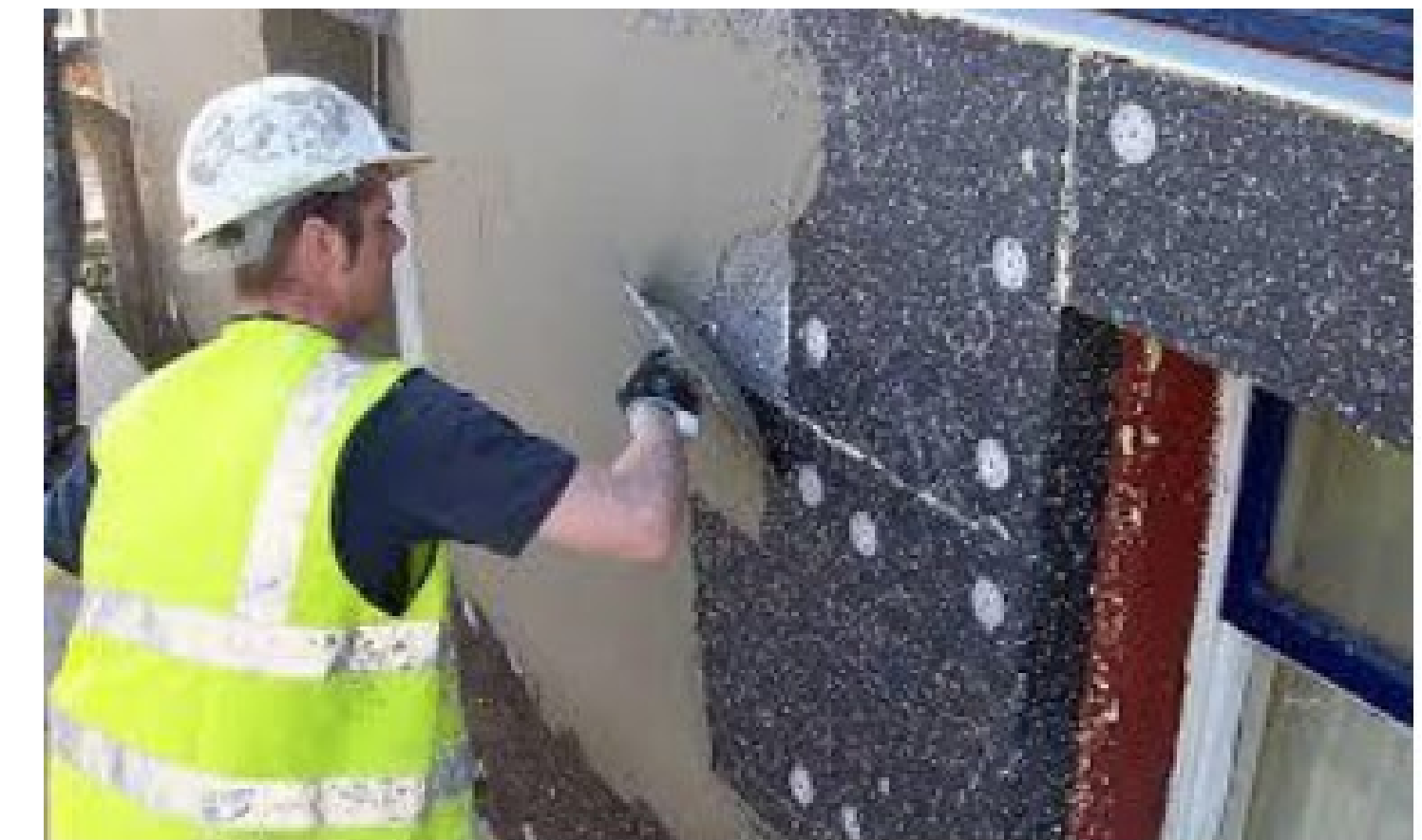
Installing Flame Retardant Foam
