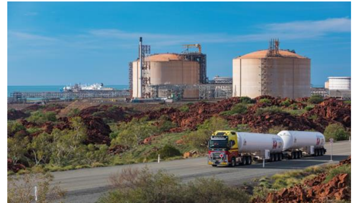
Image: LNG delivery via road train (Woodside's Pluto LNG Park and truck loading facility near Karratha in WA)
