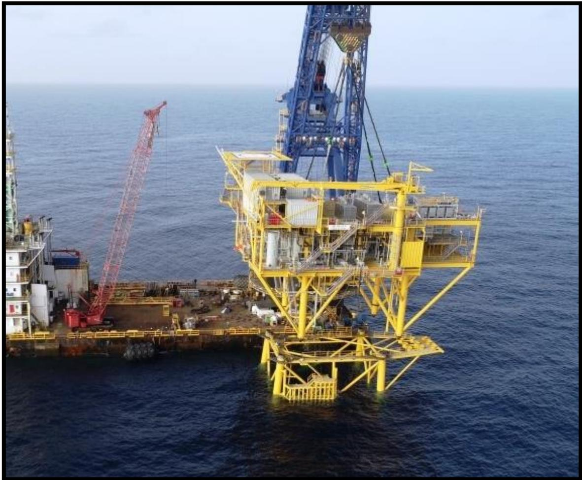
*Lifting the SM58 G Platform topside facility on to the jacket, 1 July 2020*
