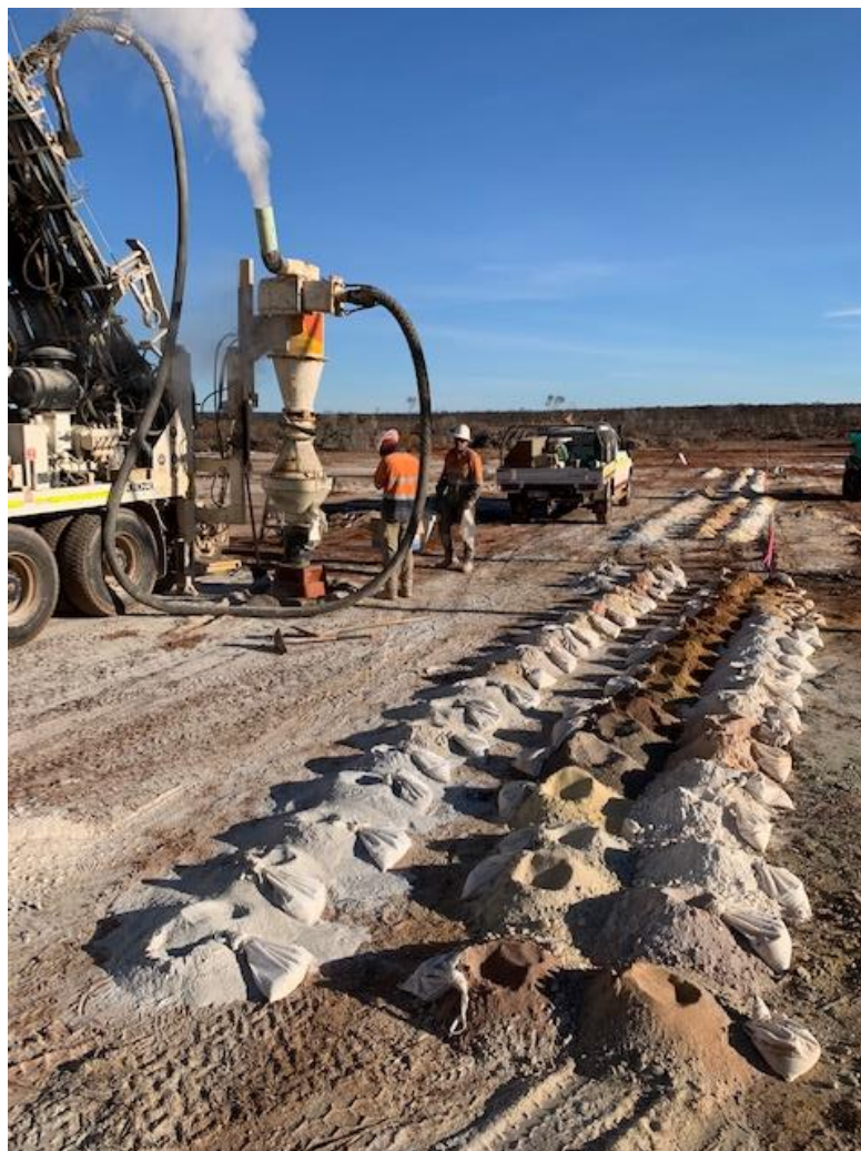
Figure 3: JUNE 2020 Drilling – Kat Gap
