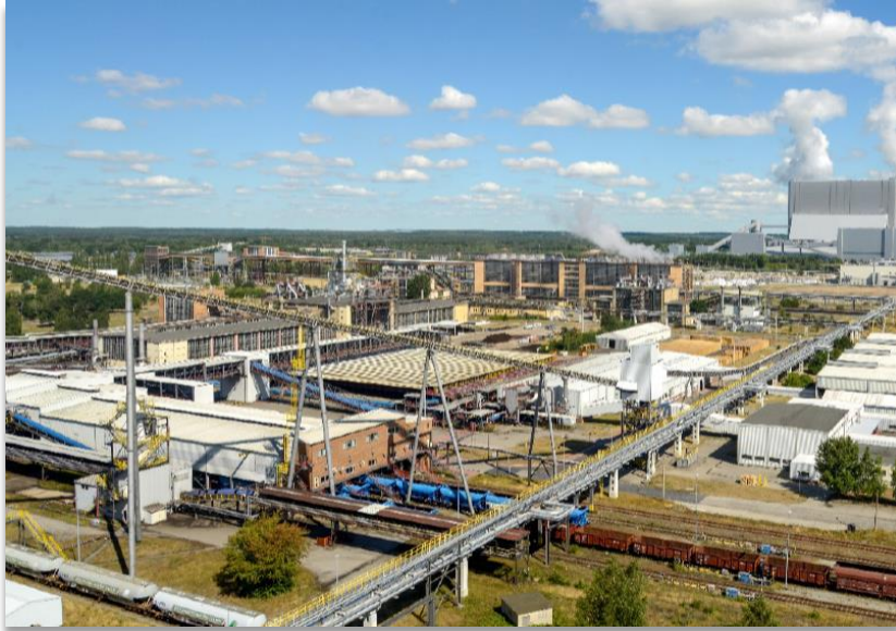
Figure 2: Schwarze Pumpe Industrial Park – showing established industry and rail line
