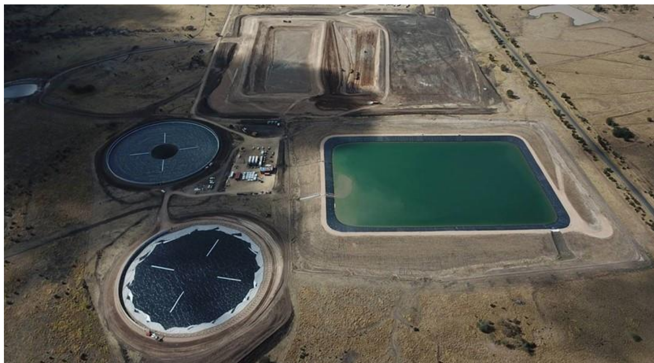
Atlas dam and water management facilities under construction
