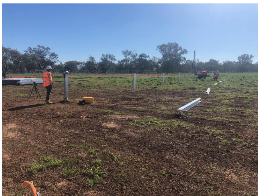
Figure 2. Piling at the Jemalong Solar Project.
