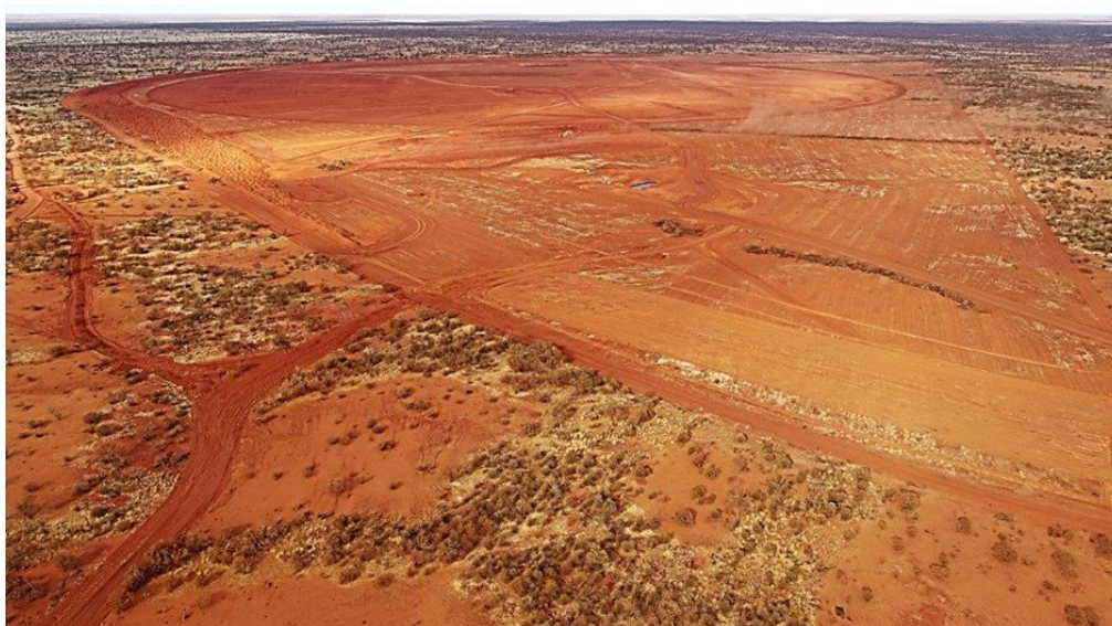
Clearing and topsoil removal for the TSF/IWL
