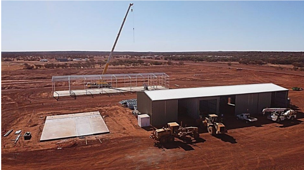
Maintenance workshop, maintenance office concrete foundation and stores shed erection
