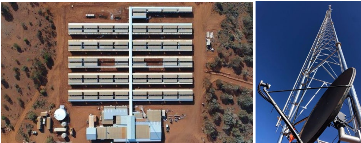
Installation of the accommodation village and communications tower
