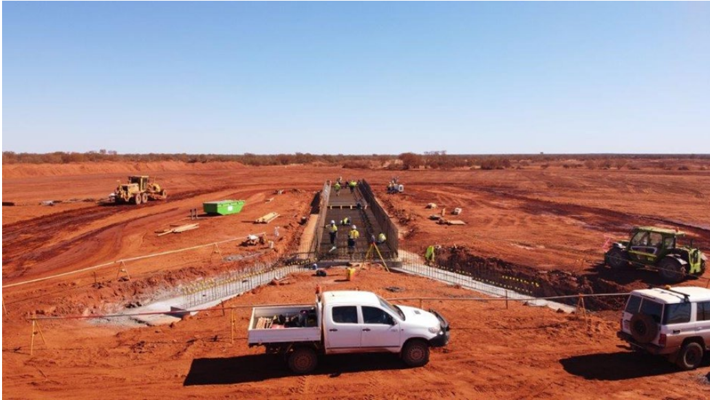
Fine ore stockpile tunnel concrete footing
