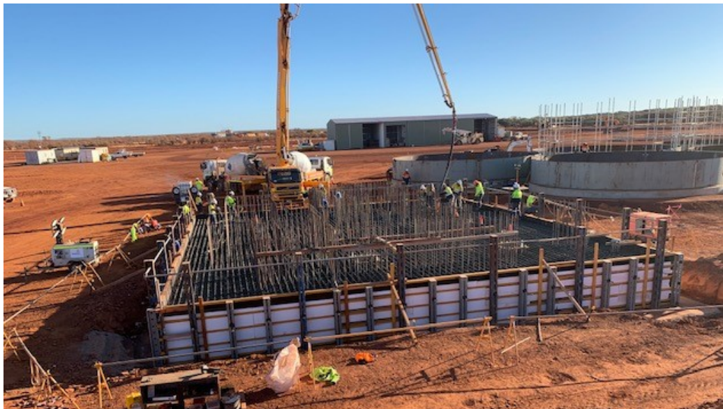
Pouring of concrete foundation for ball mill
