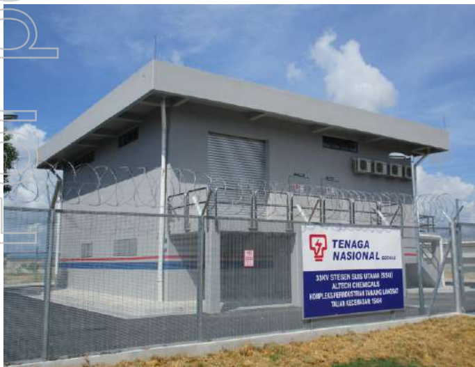
Completed electrical substation, Altech HPA plant site
