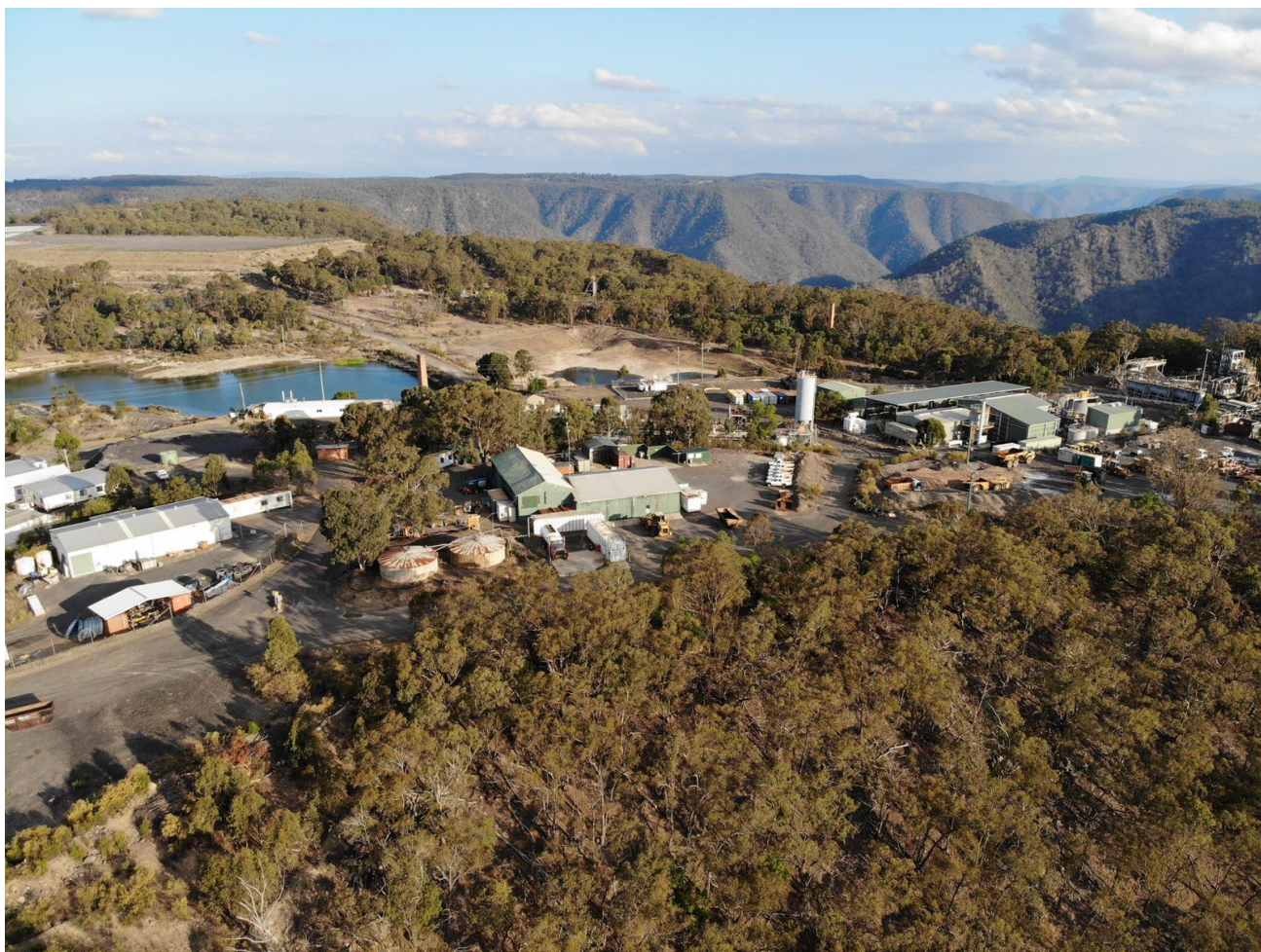
Figure 1 Hillgrove Gold Project Site, showing processing infrastructure and layout
