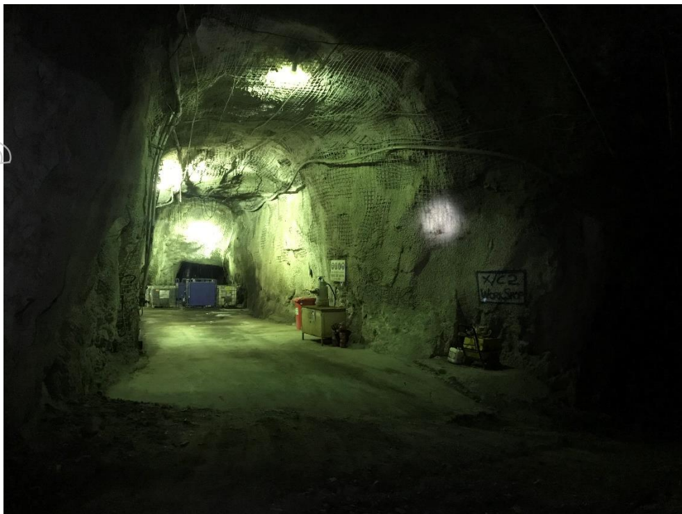
Figure 8 Metz Mining Centre UG Maintenance Workshop
