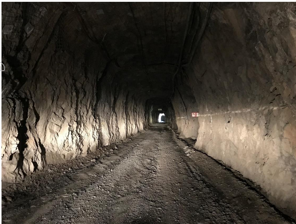
Figure 6 Metz Mining Centre Decline
