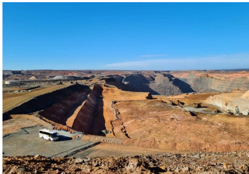
Figure 14 - Fimiston Pit, OBH cutback looking south
