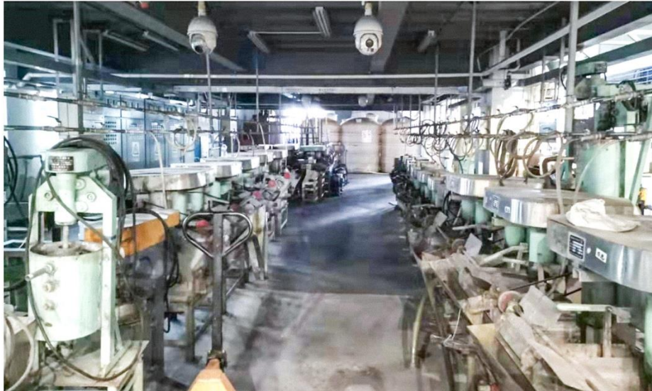
Image 5 - BGRIMM's large scale graphite pilot plant
