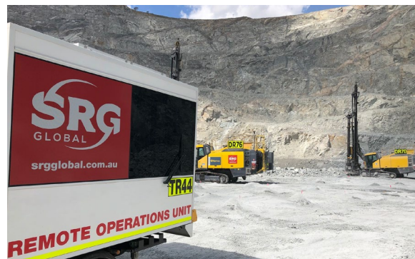
Remote Control Drilling
