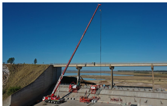
Specialist Dam Anchoring
