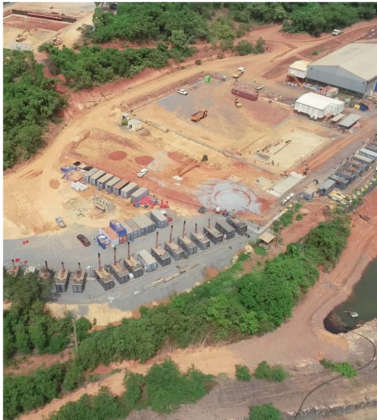
Photo: Progress at new Syama Power Plant
