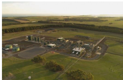
Minerva Gas Plant
