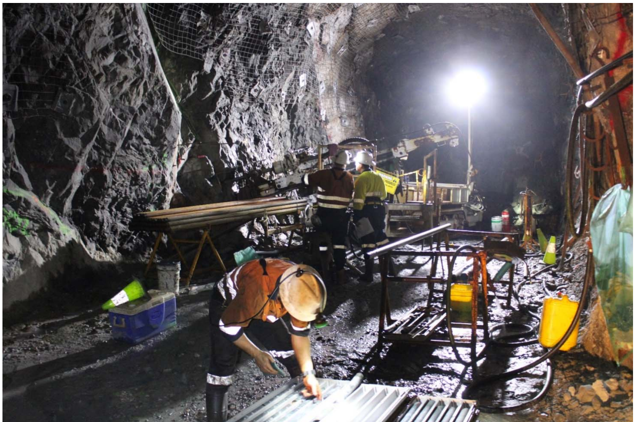
Figure 9: Underground drilling at Wiluna.
