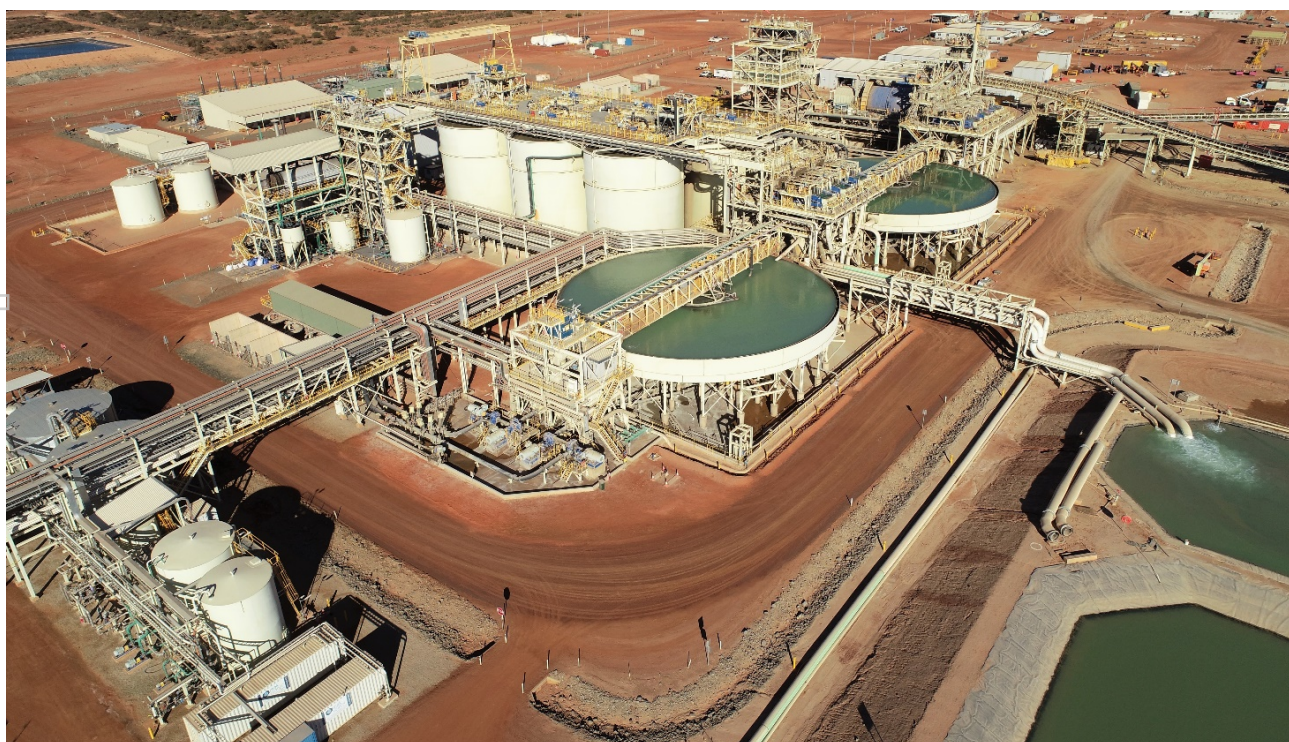
Aerial view of Process Plant
