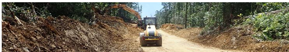
Figure 6: Construction of a road from the Wharf to the Plant site
