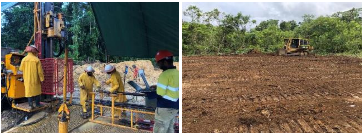
Figures 4 & 5: Geotechnical drilling program and plant site clearing works
