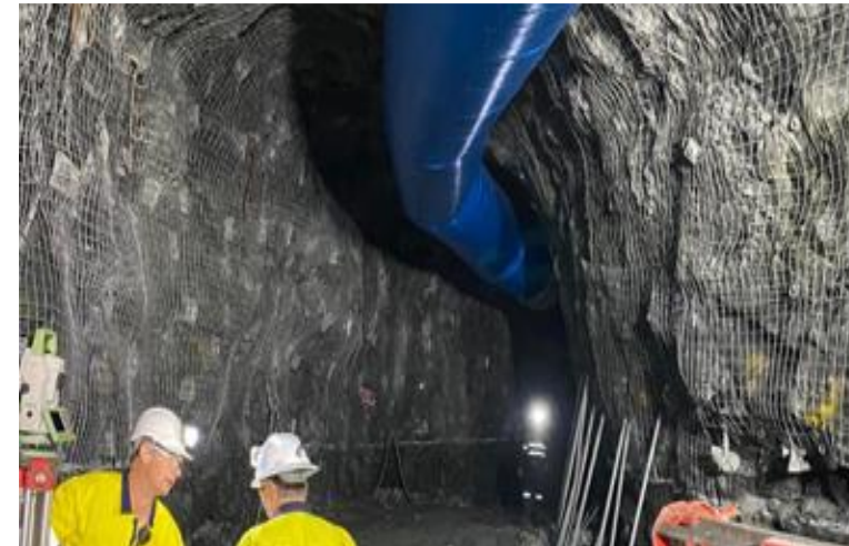
Underground development at Wiluna Mining Centre
