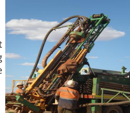
Sulphide drilling at Wiluna Mining Centre
