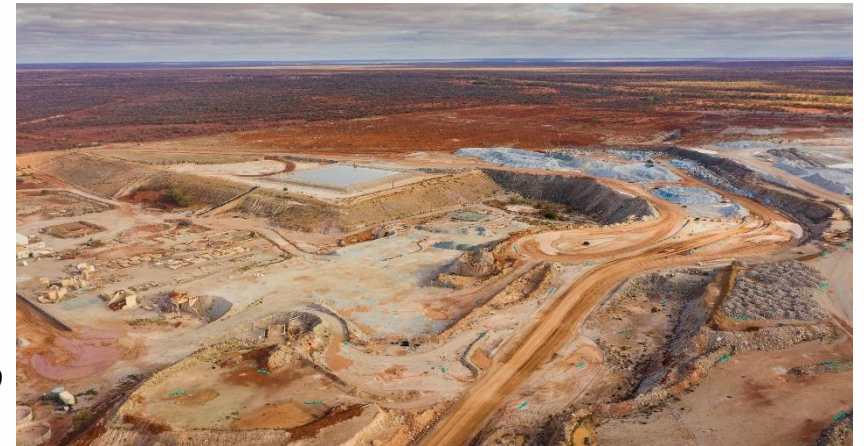
Site bulk earthworks and camp installation to start in October 2020
