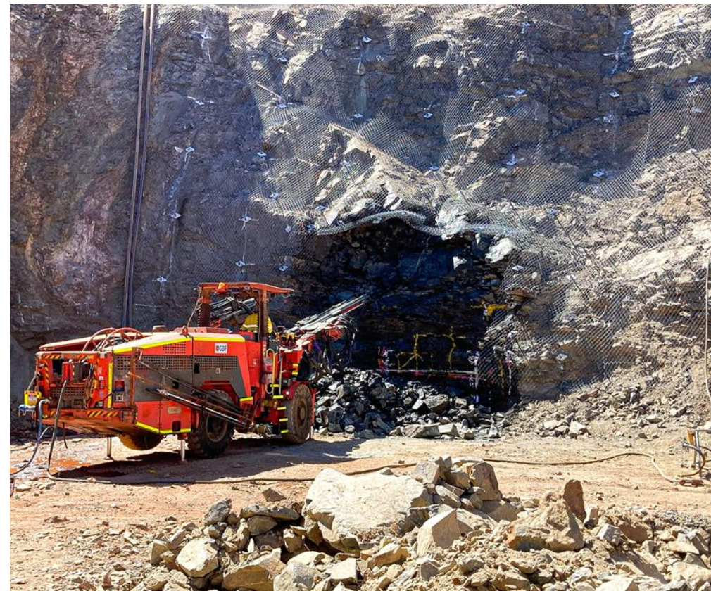
Underground portal works commencing at the Paris pit
