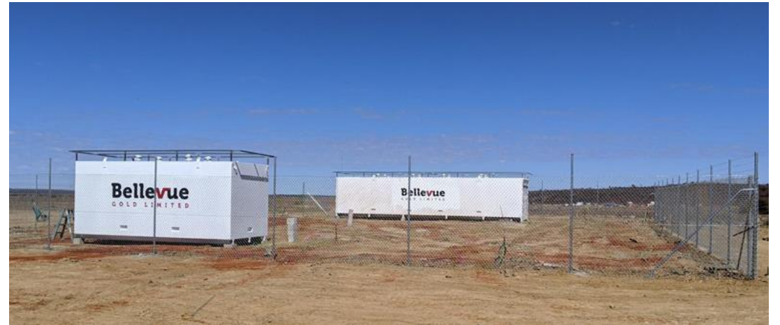
Surface Magazines being installed in preparation for underground re-entry works
