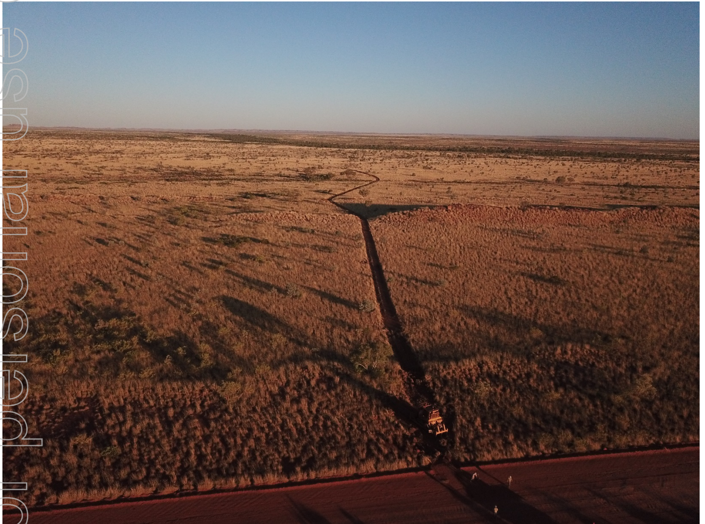
New access road construction commenced
